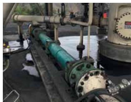
NEMO® BY Pump for the transfer of coal slurry
