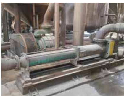
NEMO® SY pump transfers lime milk
